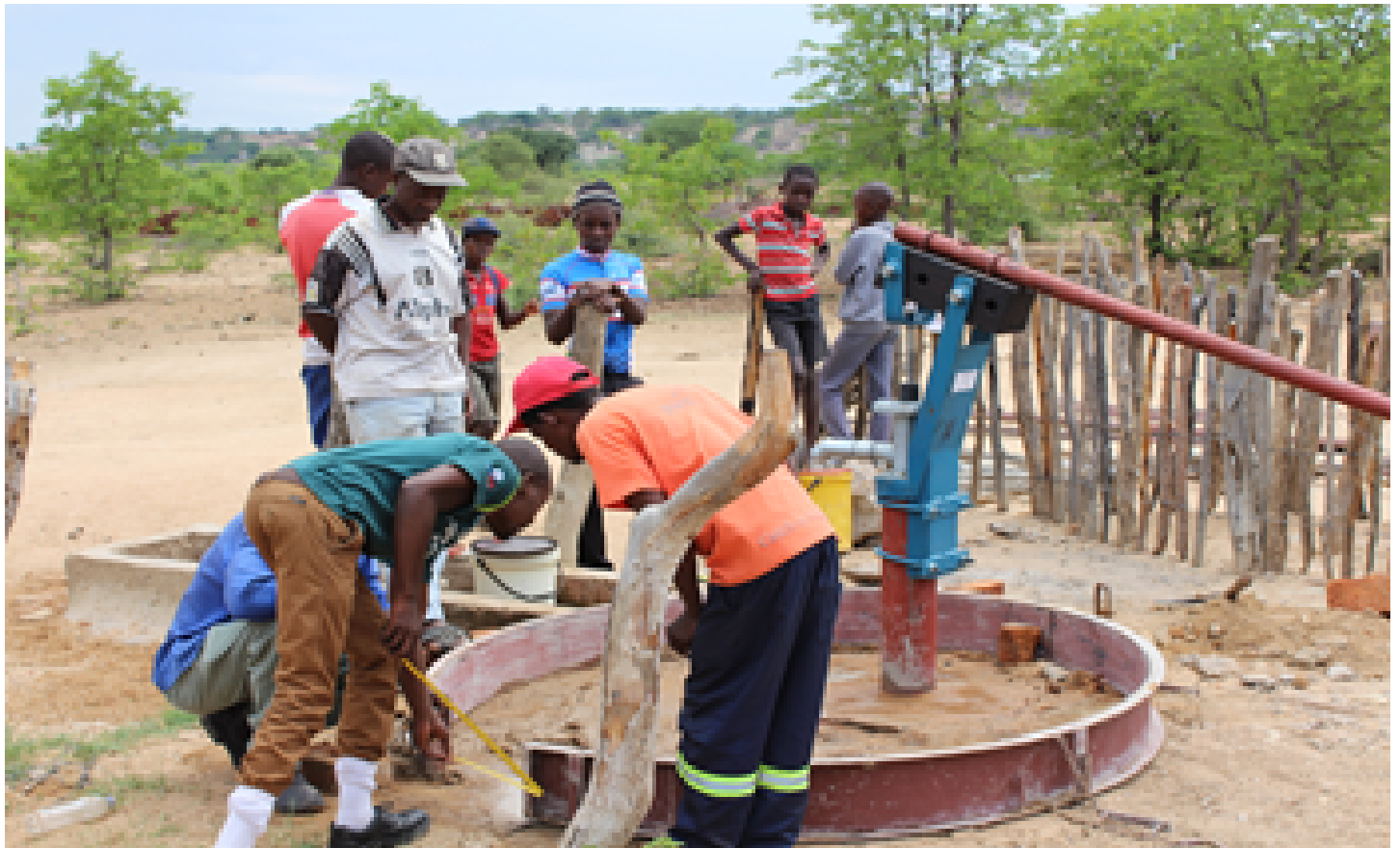
Above: Shows head works in progress in ward 4 Silawa borehole
